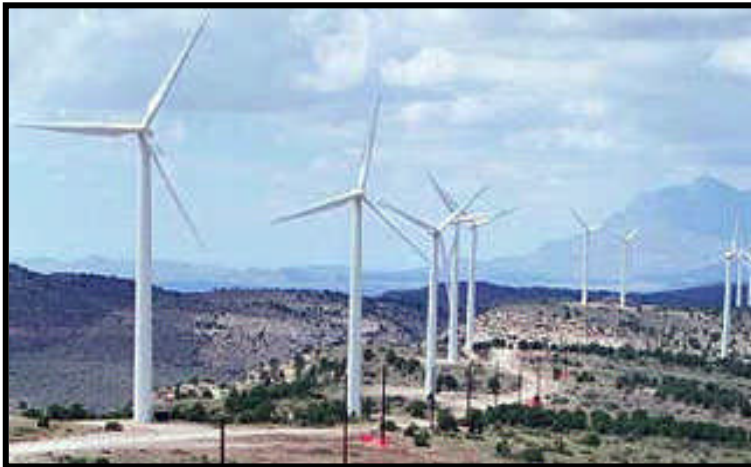
Wind Power Plant
