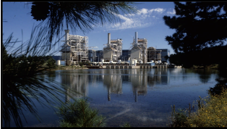
Coal, Gas, Oil-fired Steam Power Plant
