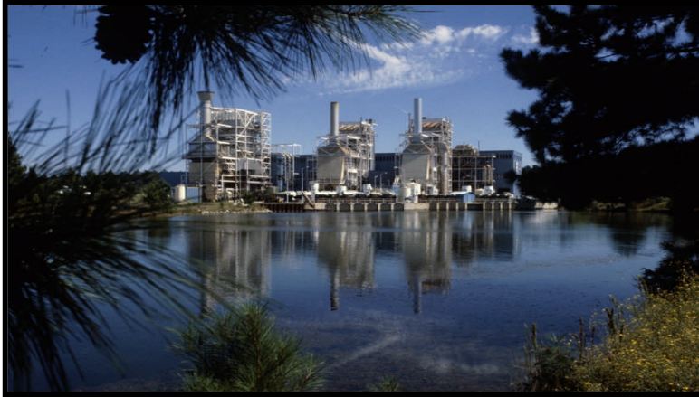
Coal, Gas, Oil-fired Steam Power Plant
