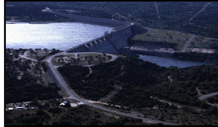
Hydro (Water) Power Plant
